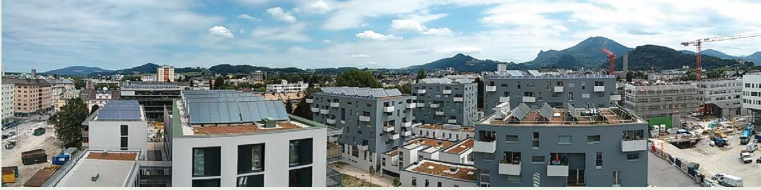
Solar thermal systems on multi-family houses in Salzburg, Austria
