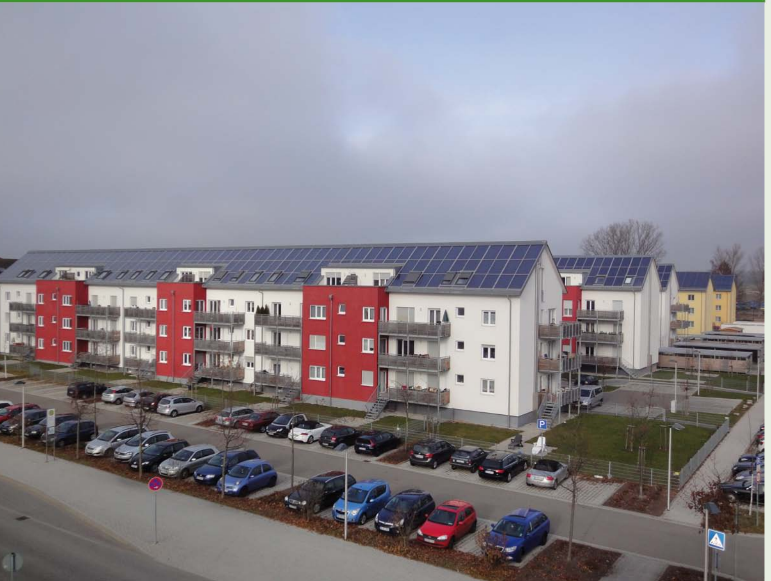
Multi-family buildings in Crailsheim, Germany. Large-scale system with 5.1 MW th installed capacity. Photo: ITW / TZS University of Stuttgart, Germany.
