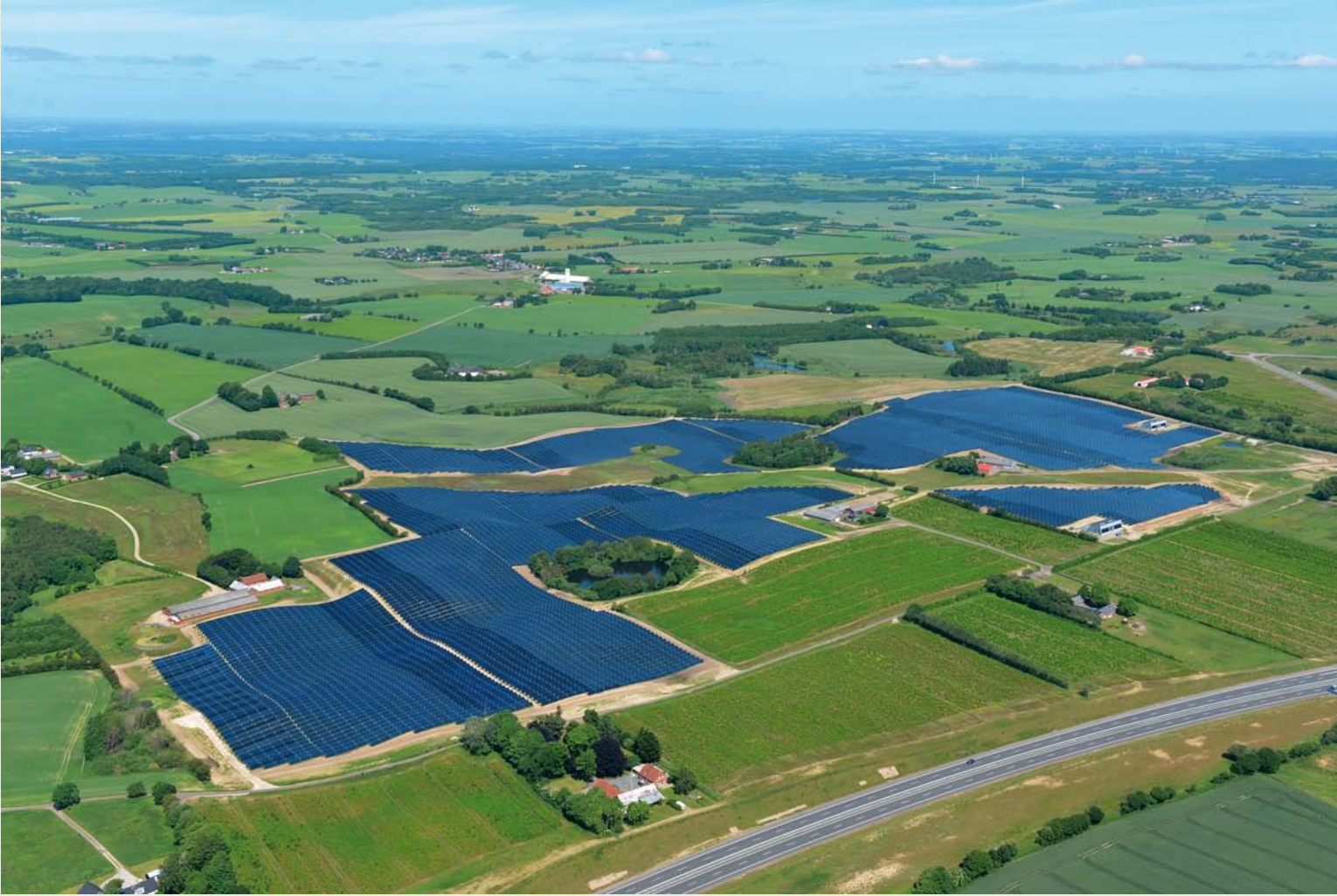
156,694 m 2 solar collector field at Silkeborg, Denmark
