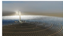
Tower solar collector
